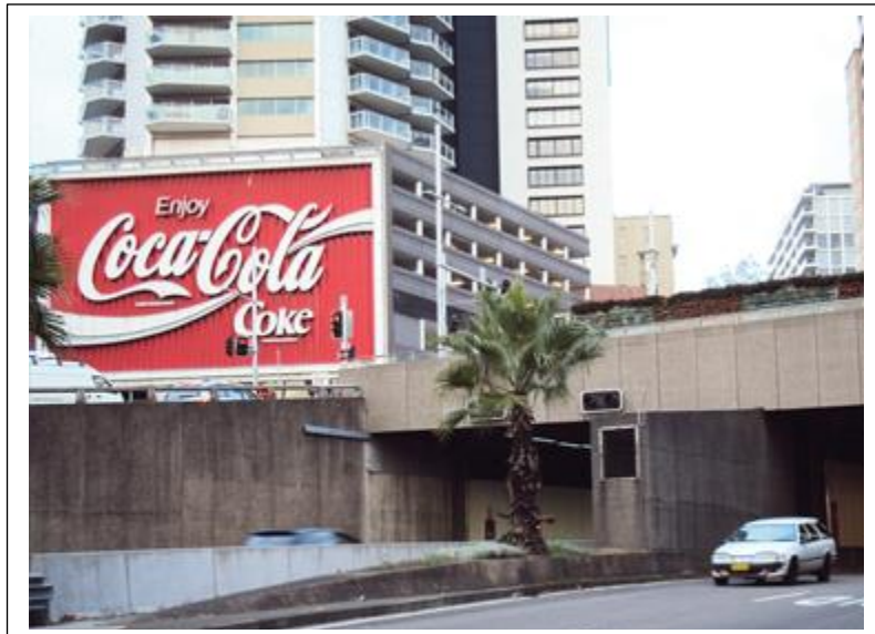
Above: Kings Cross, showing the Coca Cola sign on the corner of Darlinghurst Rd and Kings Cross Rd, the western side of the tunnel, and part of Altair at top right, built on land above the tunnel along Kings Cross Road. This road and William Street have been pathways, in various forms, for thousands of years. (Photo from www.fantech.com.au/images/Projects/kCross.jpg )
